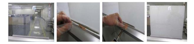
Step 12: Completely cover the bus bar area within existing frame or with Wire mold/trim (match existing finishes) to avoid exposure to electric shock. It is recommended to use a non-conductive wire mold (i.e. plastic). If you wish to use a metal wire mold we suggest you contact an electrician. Notch wire mold with dremel to accommodate wiring and attach prior to soldering. It is optional to cover remaining three edges with trim to meet any aesthetic requirements.
